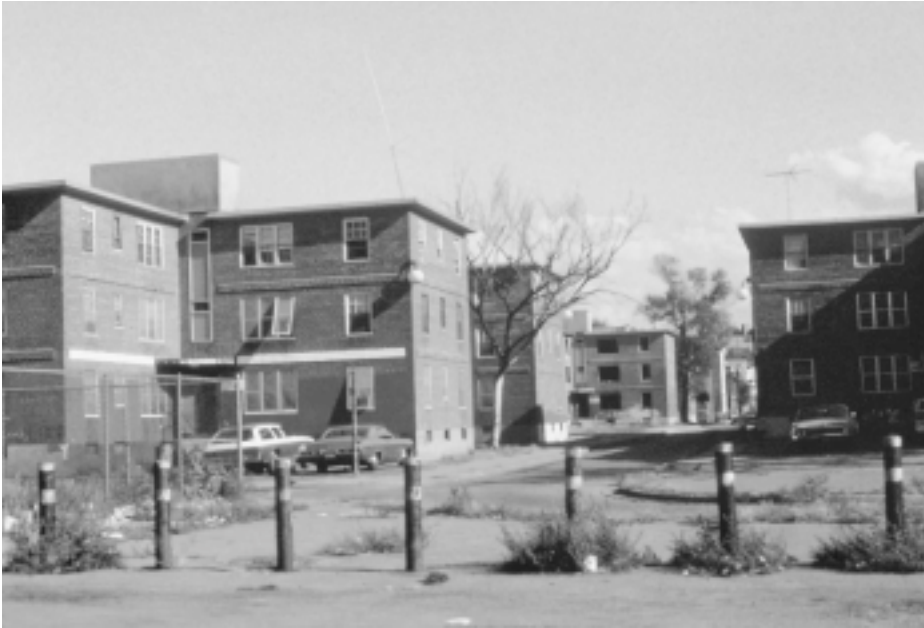
Figure 3. Site Conditions at the West Broadway Development Prior to Redevelopment (c. 1981)
