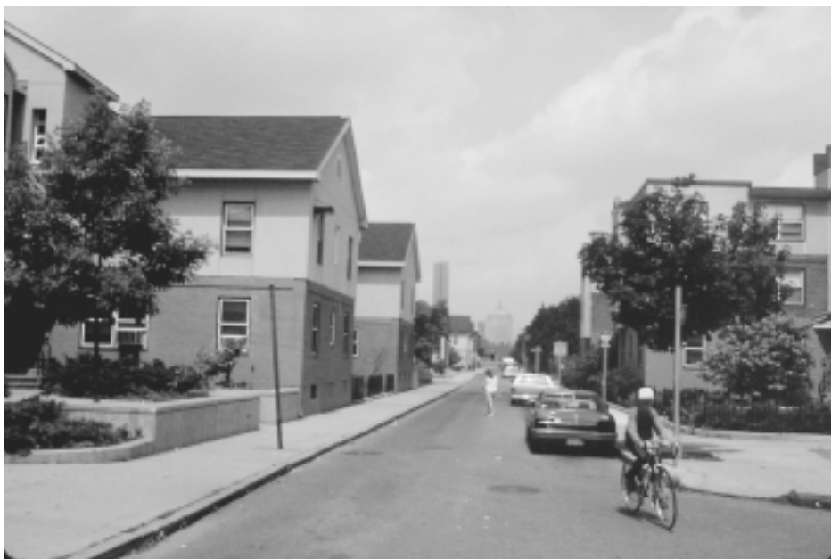
Figure 4. West Broadway Transformed
